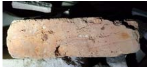
Figure 2.2. Historic common red brick used throughout the building. Note smooth surfaces and imperfections. Photo by author.
