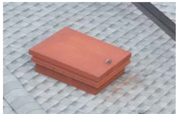
Figure 2.69. Access door on southeast facet of historic roof. Photo by author.
