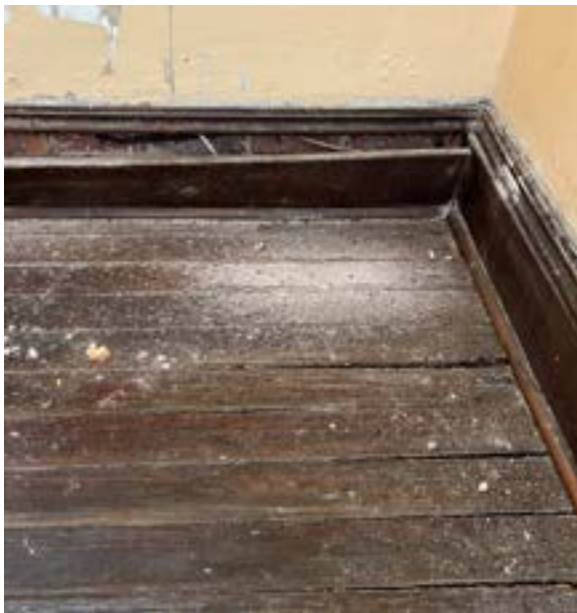
Figure 2.230. Some material failure is evident on the 2nd and 3rd platforms of the eastern stairway. Photo by author.
