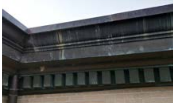
Figure 2.58. Contemporary two-piece amalgamated copper or aluminum cornice assembly. Photo by author.
