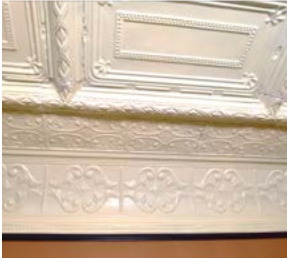
Figure 2.257. Cornice pieces are trimmed with small wood molding. Photo by author.
