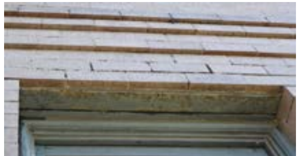
Figure 2.126. Steel lentiil above larger historic windows. Photo by author.
