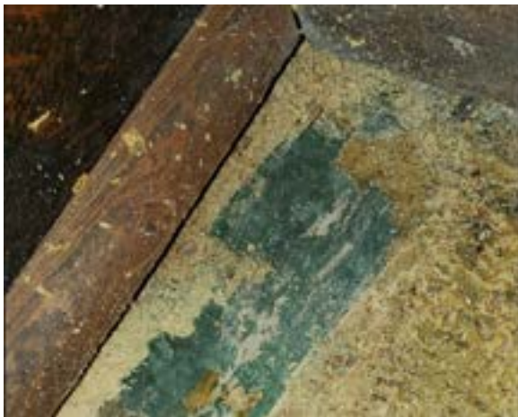
Figure 2.234. Hard density tile flooring located behind circulation desk is likely an asbestos product and should be approached and handled according to local and state abatement requirements. Photo by author.
