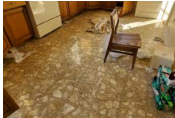
Figure 2.240. Vinyl flooring in kitchen. Photo by author.
