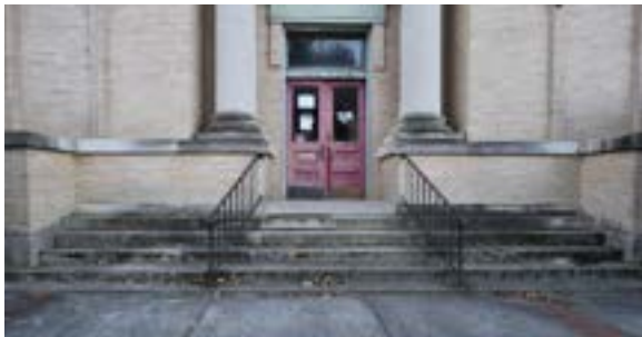
Figure 2.183. Main entry stairs rise 37" above sidewalk grade. Photo by author.
