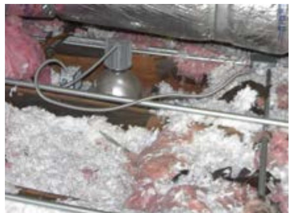
Figure 2.284. More recent electrical wiring housed in EMT (rigid and flexible). Photo by author.
