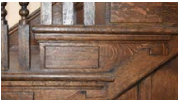
Figure 2.228. Outer stringer detailing. Photo by author.
