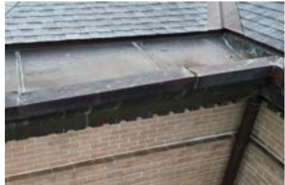
Figure 2.54. Box gutter assembly on historic building (northwest corner). Photo by author.
