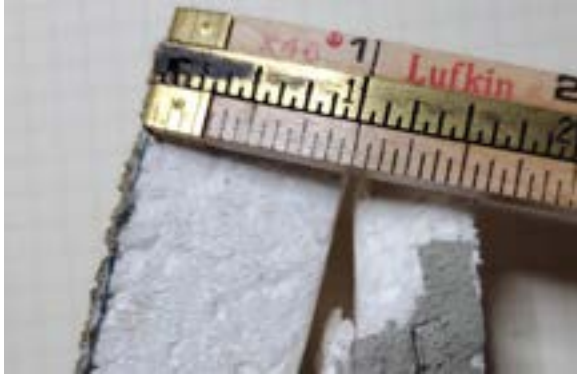
Figure 2.108. Two sheets of 1" EPS were installed. Photo by author.
