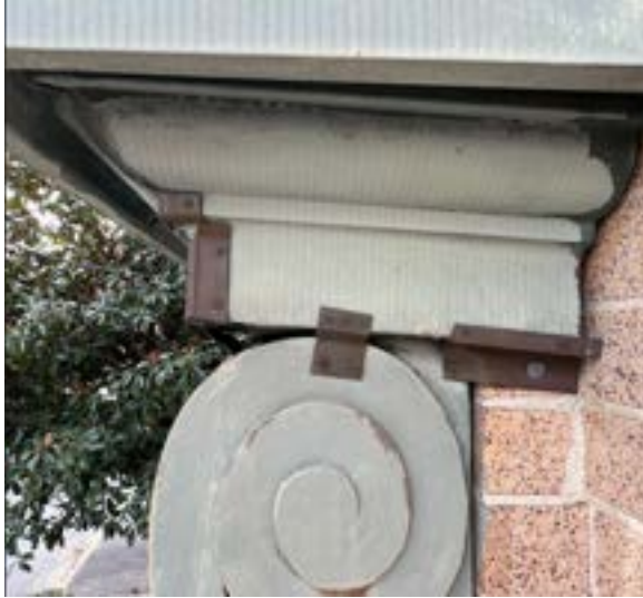
Figure 2.155. Excellent and stable repairs to HO5 & HO6. Photo by author.
