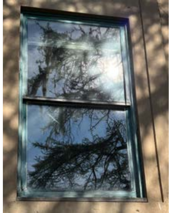
Figure 2.131. A double sash window in the modern addition. Photo by author.
