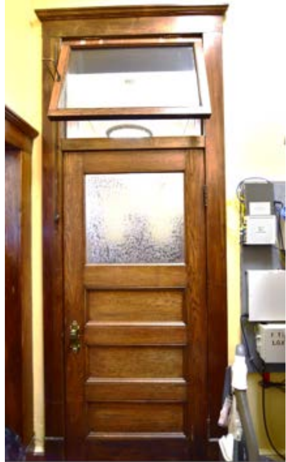
Figure 2.172. All mechanisms on librarian doors are functional. Photo by author.
