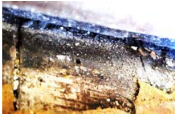
Figure 2.236. Wood flooring below first floor carpet. Photo by author.
