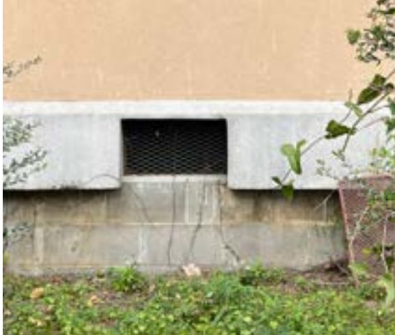
Figure 2.27. Six foundation windows below modern addition. Photo by author.
