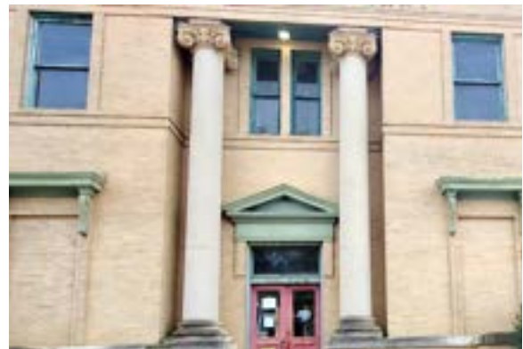
Figure 2.92. Building entry framed by monumental limestone columns. Photo by author.
