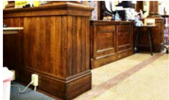
Figure 2.220. All columns sit on wainscot wrapped piers. Photo by author.
