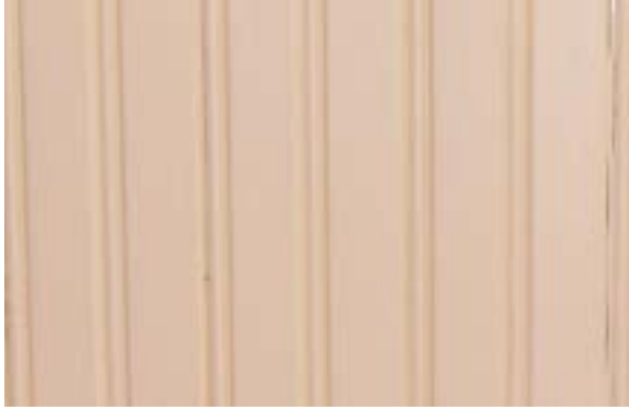
Figure 2.261. Beadboard ceiling on second floor. Photo by author.
