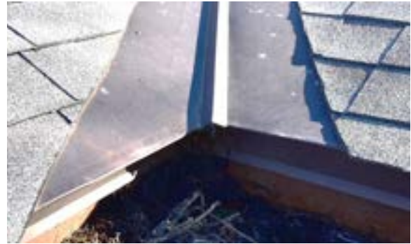
Figure 2.72. Close-up of copper valley flashing. Photo by author.
