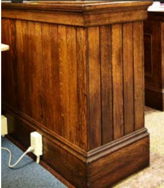
Figure 2.200. Wainscoting covers the perimeter of the interior first floor walls. Photo by author.
