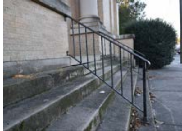
Figure 2.184. Non-historic handrail. Photo by author.
