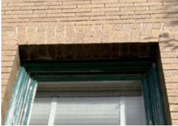
Figure 2.127. A masonry jack arch above narrower windows. Photo by author.
