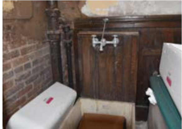
Figure 2.305. Surviving water faucet and basin below eastern stairway. Photo by author.
