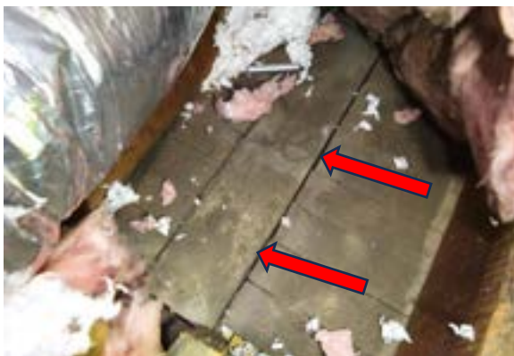
Figure 2.31. Original 2" x 6" top plate of kitchen demising wall in attic. Photo by author.
