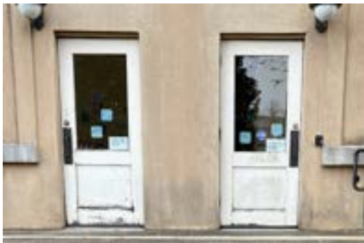
Figure 2.166. ADA compliant doors on west side of addition. Photo by author.
