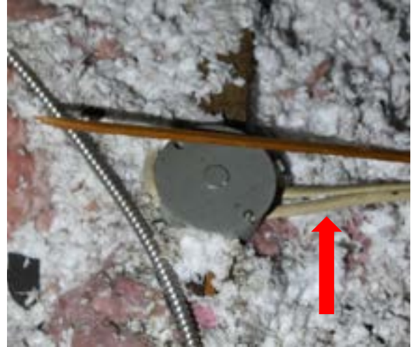
Figure 2.283. Modern Romex wiring in evidence throughout building. Photo by author.
