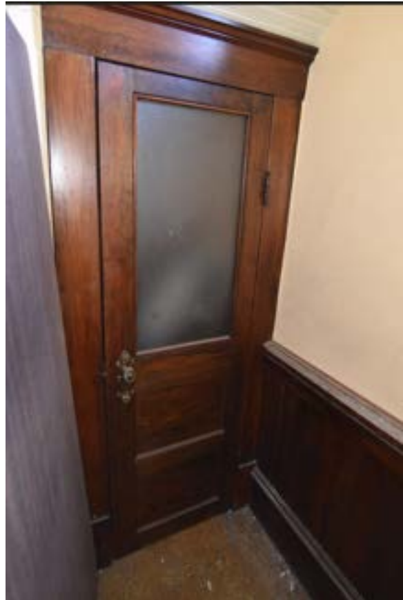
Figure 2.223. The hidden bathroom door below western foyer stairs. Photo by author.
