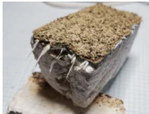
Figure 2.107. EIFS Sample from addition exterior wall. Photo by author.
