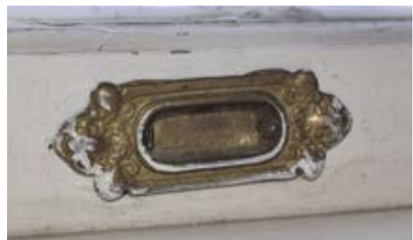
Figure 2.123. Hardware on historic windows. Photo by author.
