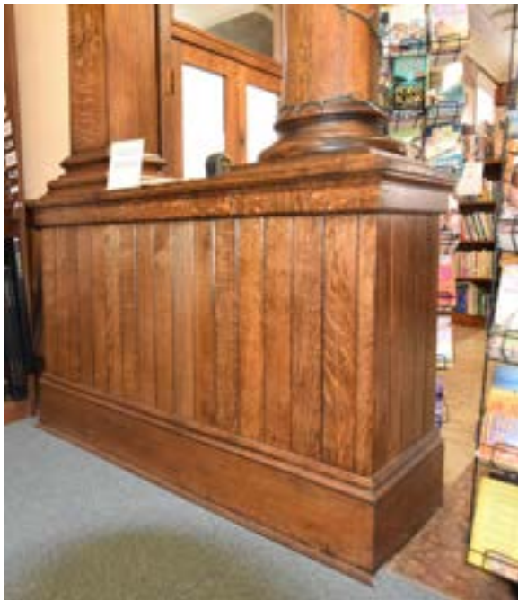
Figure 1.70. Interior oak detailing includes wainscoting, trim, columns, and doors. Photo by author.
