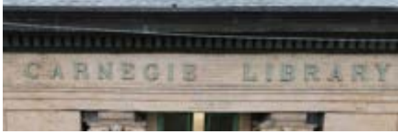
Figure 2.97. Wall culminates with dentil molding and cornice. Photo by author.
