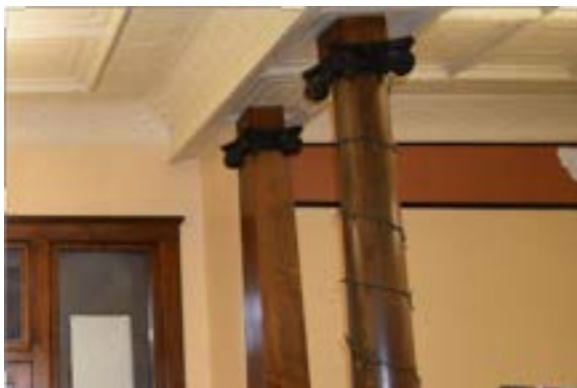
Fig. 2.218. Box columns are engaged with the wall. Photo by author.
