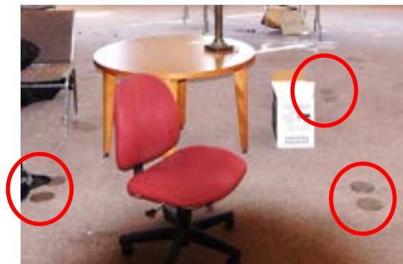
Fig. 2.287. Access caps for LED light upgrade location on second story floor. Photo by author.
