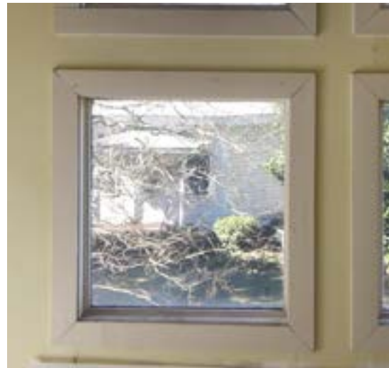
Figure 2.139. Miter corners on casement windows. Photo by author.
