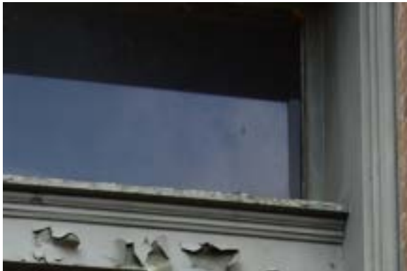
Figure 2.159. Main entrance transom window. Photo by author.
