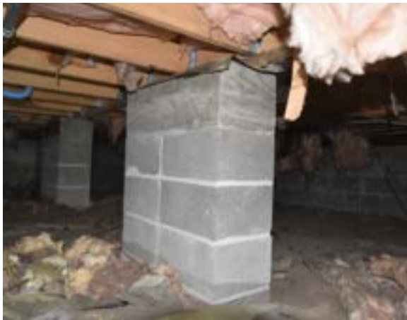
Figure 2.28. CMU piers supporting flooring system of addition. Photo by author.
