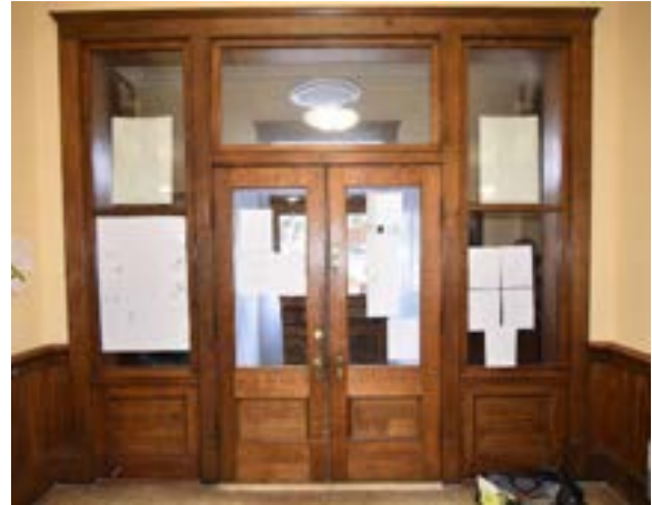
Figure 2.167. Main entryway inside first floor. Photo by author.
