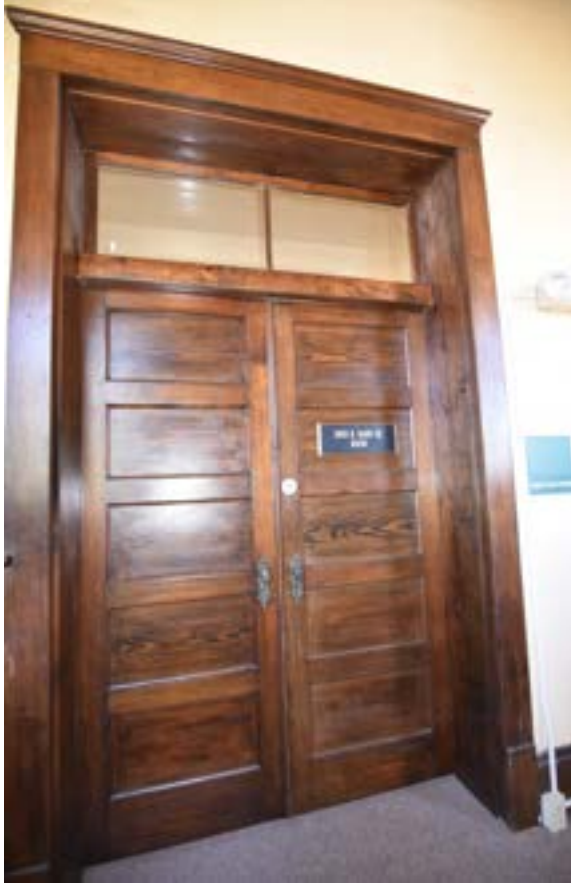
Figure 2.168. Western pair of two entryways on second floor. Photo by author.
