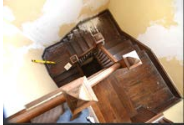
Figure 2.225. The stairs are configured as three-quarter winders. Photo by author.
