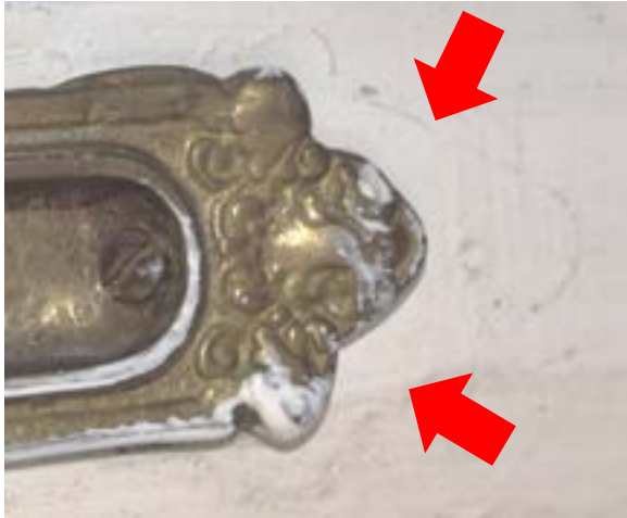
Figure 2.124. Evidence of prior hardware set observed on most lower sashes. Note ghosted outline highlighted by red arrows. Photo by author.
