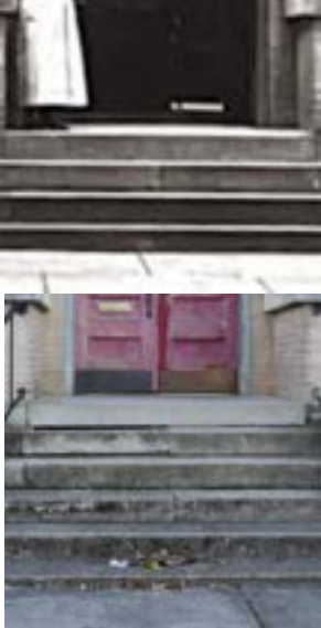
Figure 2.158 Two steps were added at bottom of main entrance stairway, notice difference from historic configuration pictured above.
