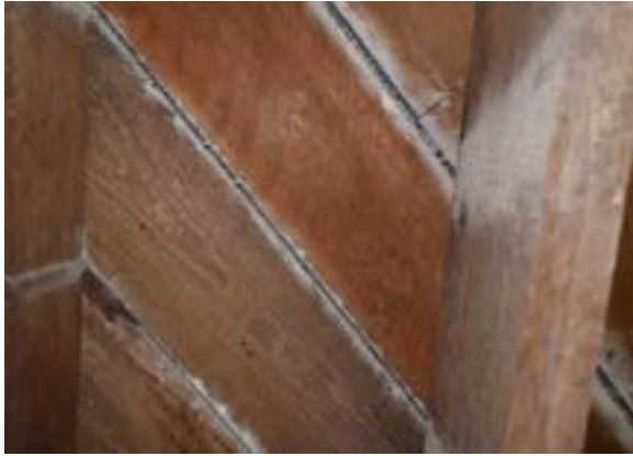
Figure 2.37. The subfloor is 1" x 8" (nominal) laid diagonally. Photo by author.
