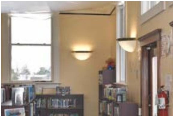
Figure 2.201. Approximately 50% of the interior walls are drywall with taped and sanded seams. Photo by author.
