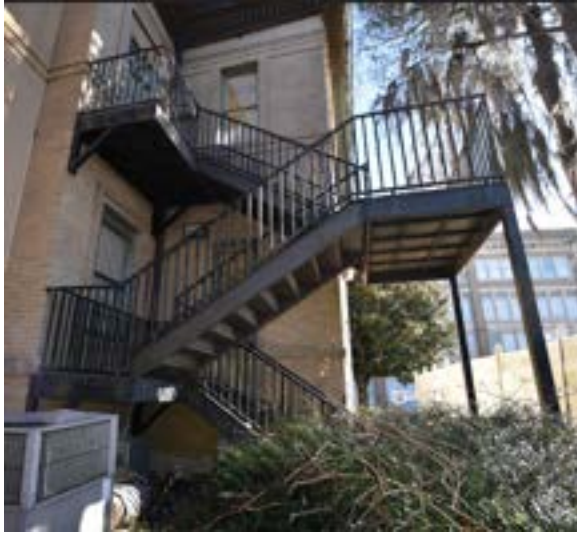
Figure 2.186 Fire escape on south side of building. Photo by author.
