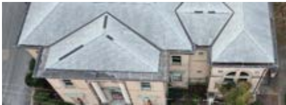
Figure 2.56. Note different distances box gutter projects off building. Photo by author.
