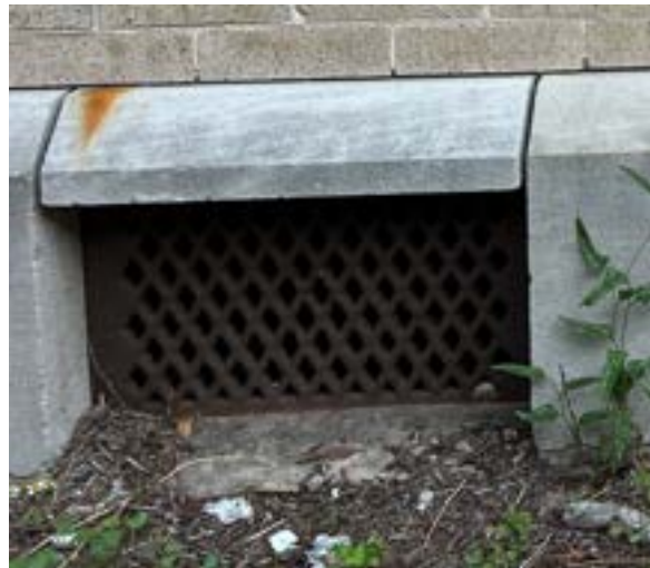
Figure 2.7. Historic building foundation windows. Photo by author.
